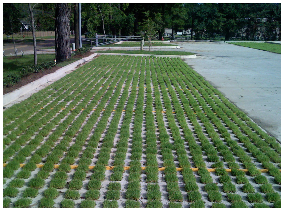
Pervious paving system absorbs rainfall and reduces heat
