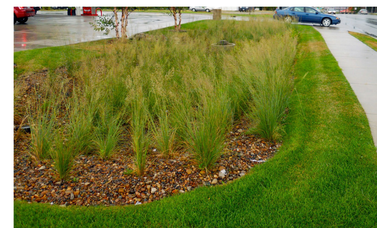
Planted bioswales within the block store water during rain events.
