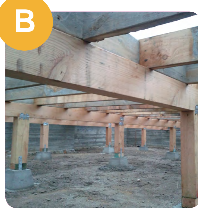
Pier and Beam Foundations
