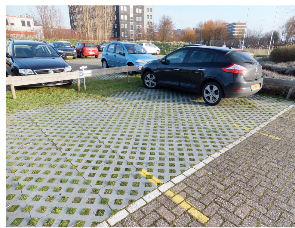
Pervious pavers in parking spaces help to absorb rainfall runoff.
