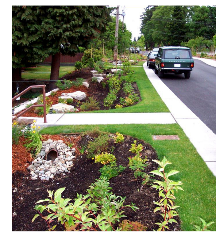
Perimeter bioswales are planted with native plants. During wet conditions curb cuts allow water to run off from the streets into bioswales.
