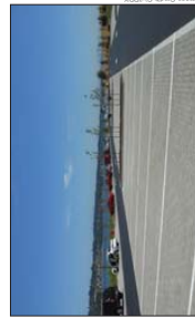
Permeable pavement allows rainwater through at Gleason Boat Ramp, Portland, OR.
