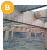
Pier and Beam Foundations
