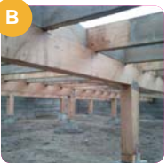
Pier and Beam Foundations
