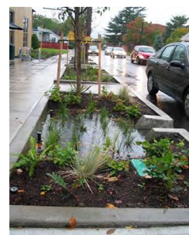
Perimeter bioswales are planted with native plants. During wet conditions curb cuts allow water to run off from the streets into bioswales.
