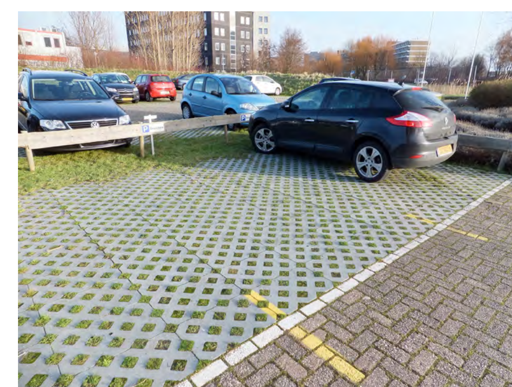
Pervious pavers in parking spaces help to absorb rainfall runoff.
