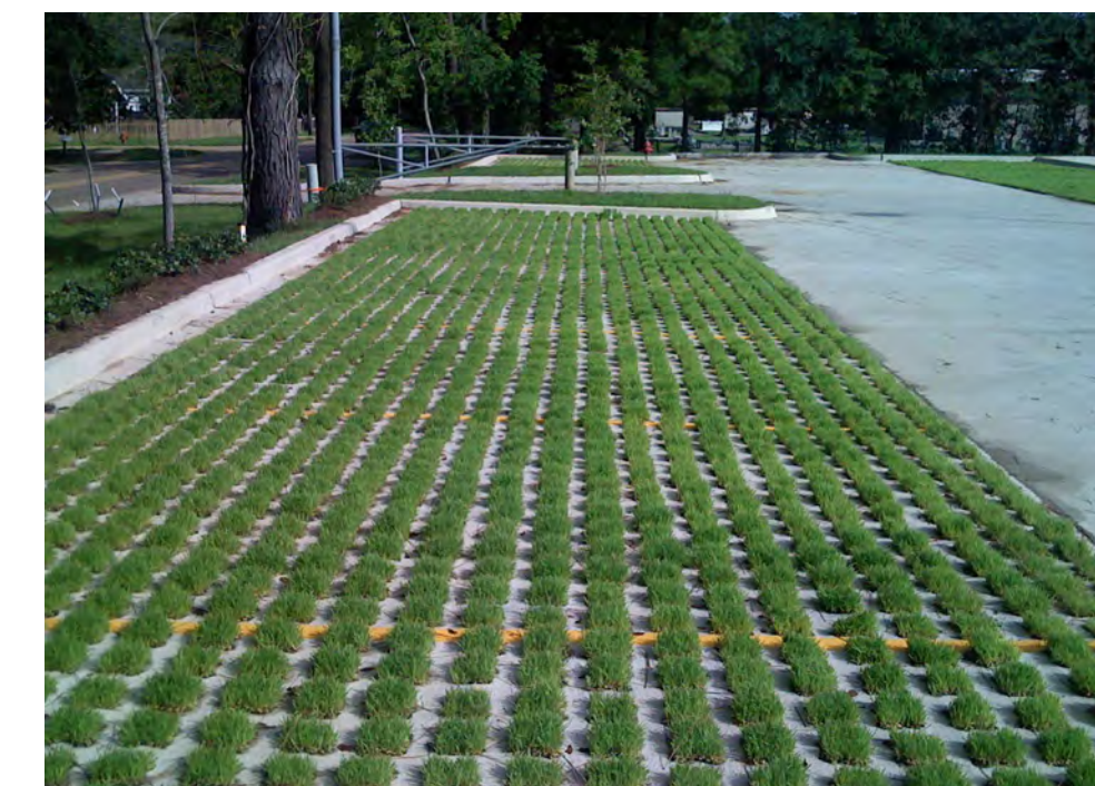
Pervious paving system absorbs rainfall and reduces heat
