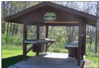
Fish cleaning station at Blackhawk Lake Recreation Area, Highland, WI.
