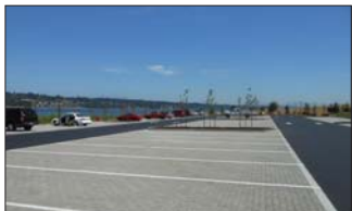
Permeable pavement allows rainwater through at Gleason Boat Ramp, Portland, OR.
