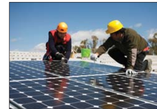
Solar panel installation
